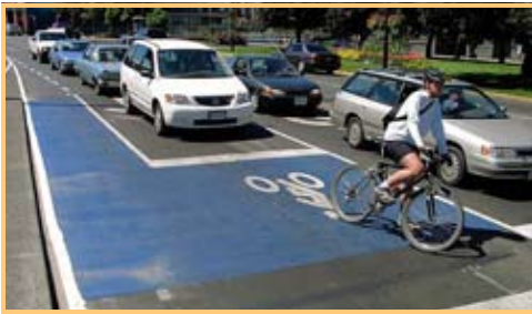
In-line bike box makes left turns easier
