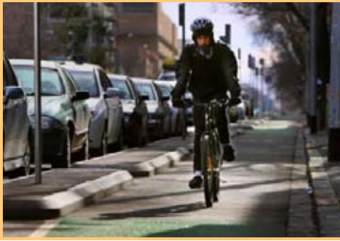
Separated bike lane next to parking
