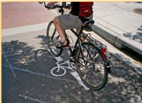
Bike-activated traffic signal
