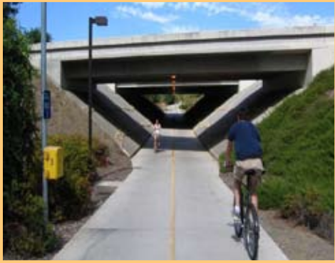
Underpass beneath arterial road
