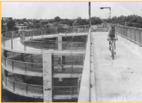
Spiral ramp bridge crosses highway
